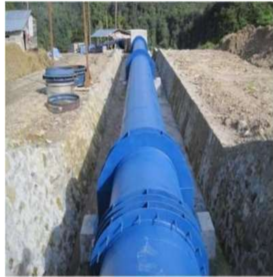
Gambar 3. Pipa pesat ( penstock )
